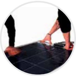
6. After pasting, it is very important to apply pressure on the whole bonded surface. For this purpose it may be sufficient treading repeatedly the module itself, so as not to leave parts not subject to foot traffic, of course, taking care not to use too rigid and angular footwear.
