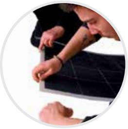
5. Now, install starting on the one hand by joining form in a progressive manner to prevent the formation of air bubbles (for any doubts consult our website).
